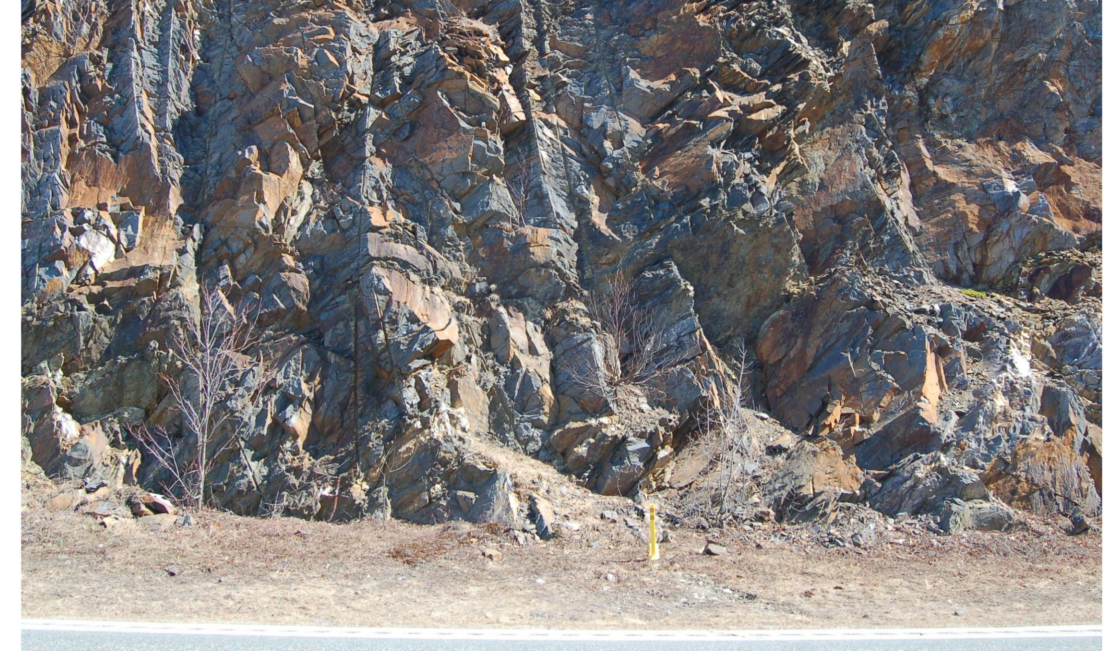
STA. 1855+00 MACHINE SCALING AT TOP ONLY
