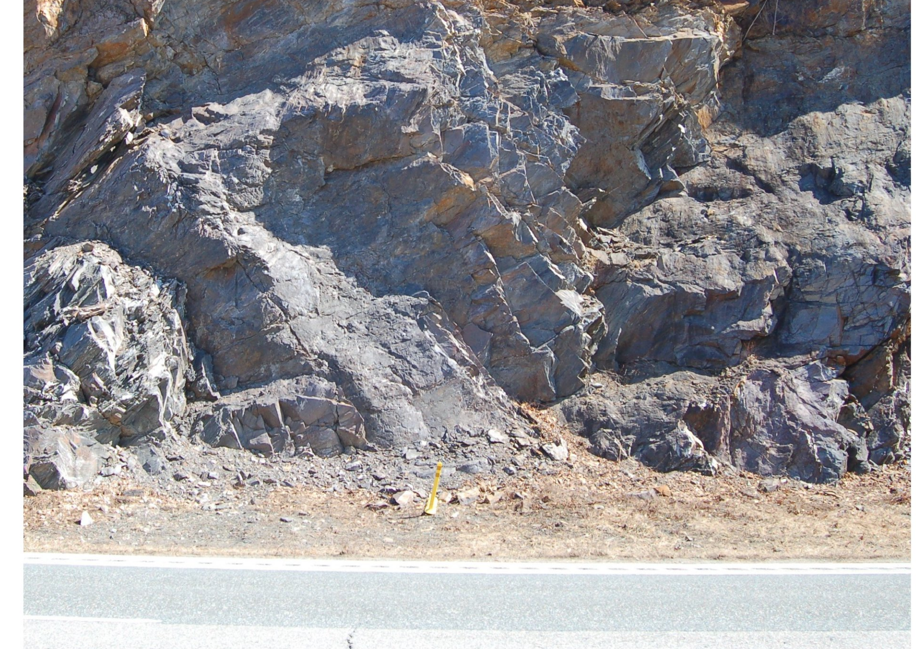
STA. 1849+00 MACHINE SCALING AT TOP ONLY
