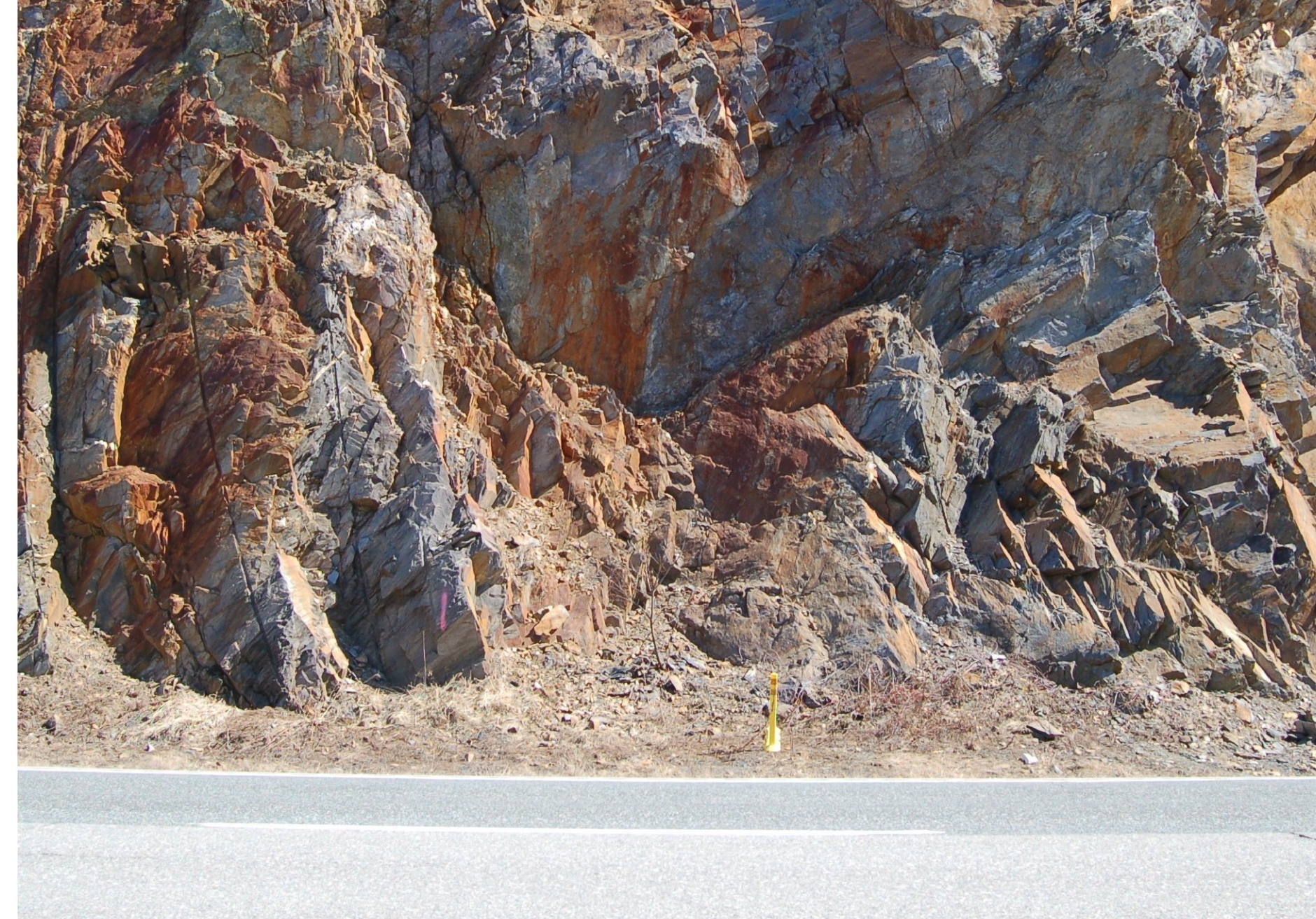
STA. 1853+50 MACHINE SCALING AT TOP ONLY
