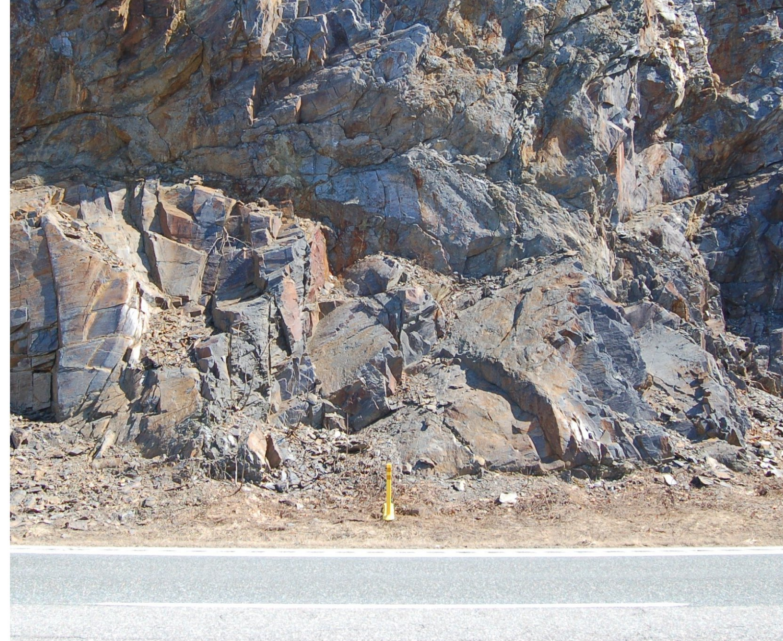
STA. 1851+50 MACHINE SCALING AT TOP ONLY
