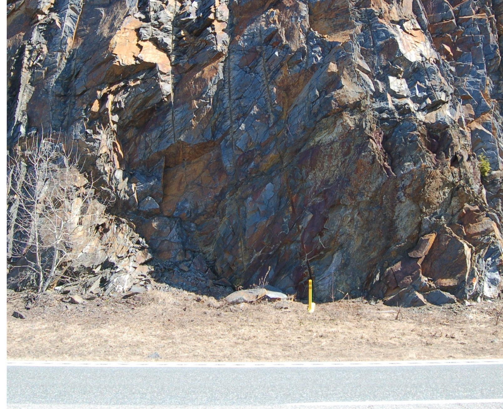
STA. 1856+00 MACHINE SCALING AT TOP ONLY
