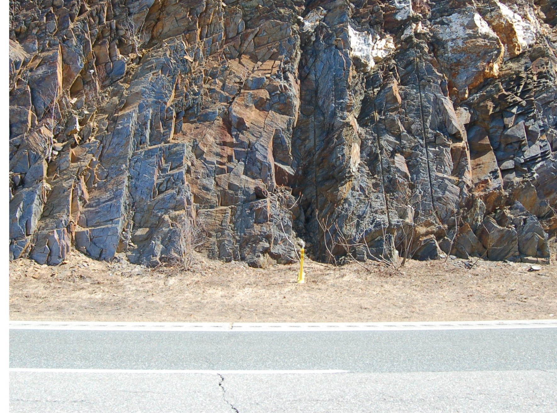
STA. 1857+50 MACHINE SCALING AT TOP ONLY
