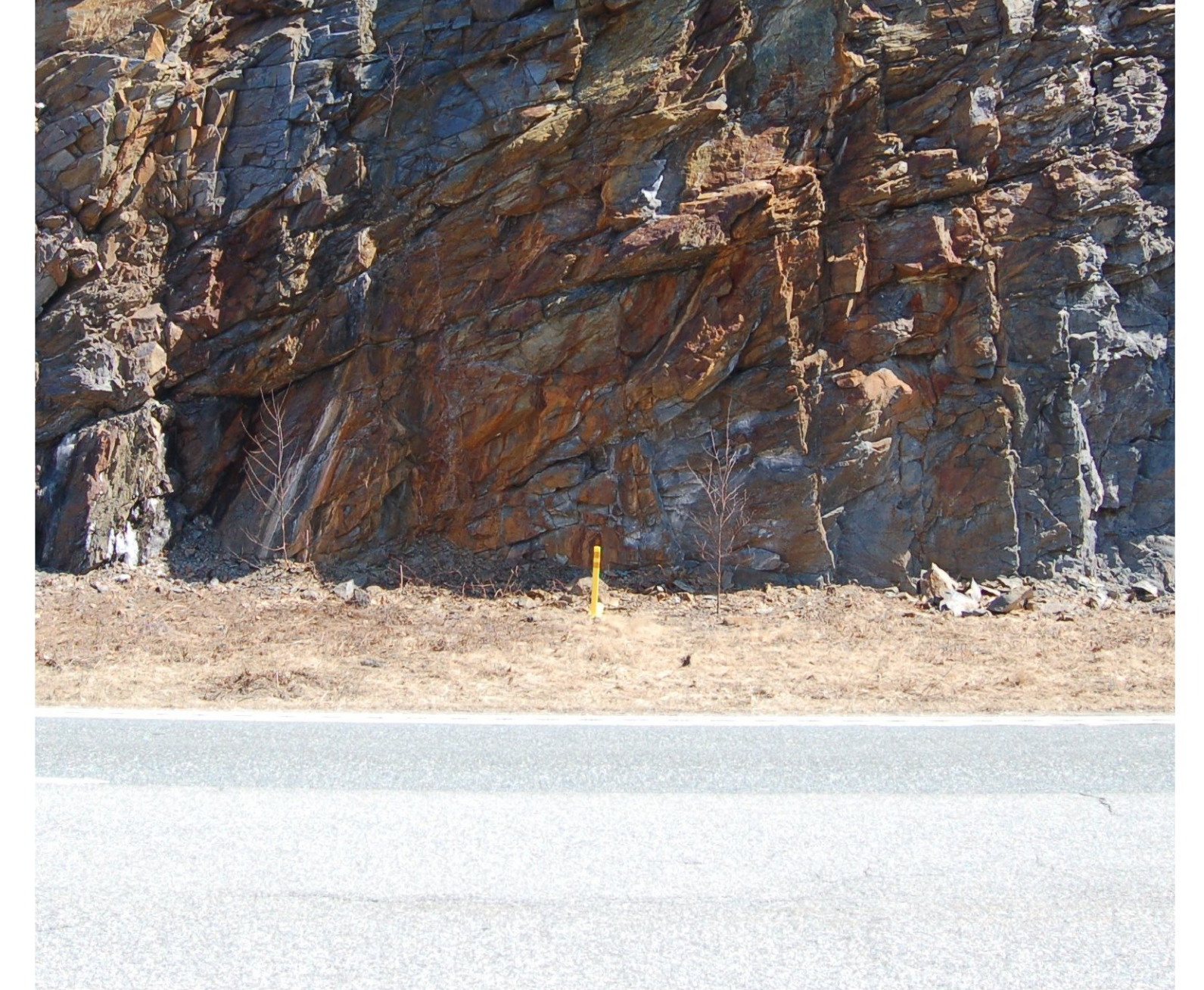
STA. 1847+00 MACHINE SCALING AT TOP ONLY
