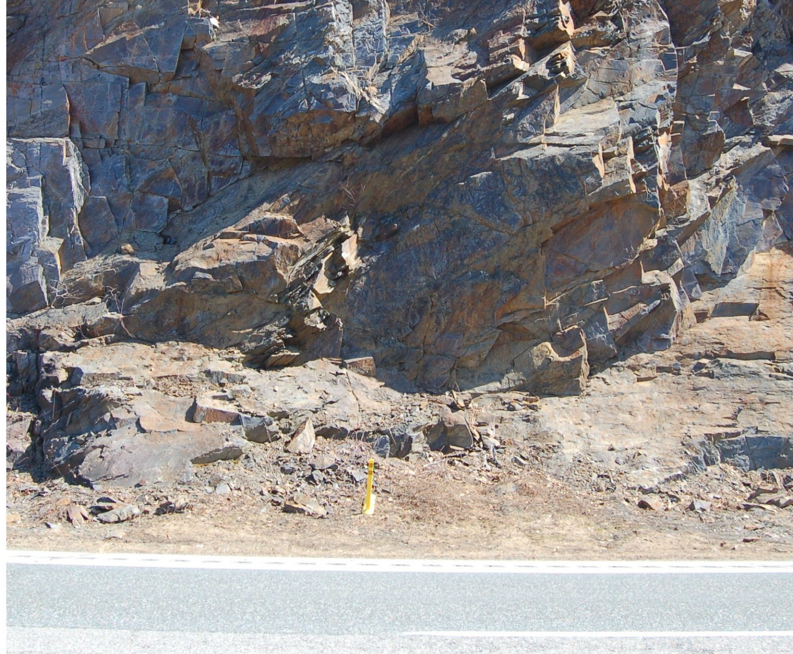
STA. 1850+00 MACHINE SCALING AT TOP ONLY
