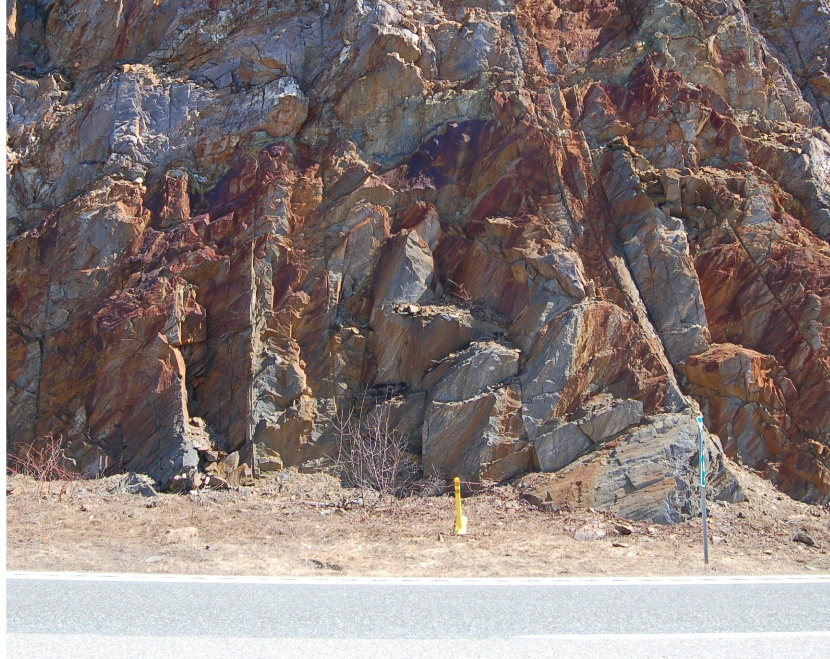
STA. 1854+00 MACHINE SCALING AT TOP ONLY
