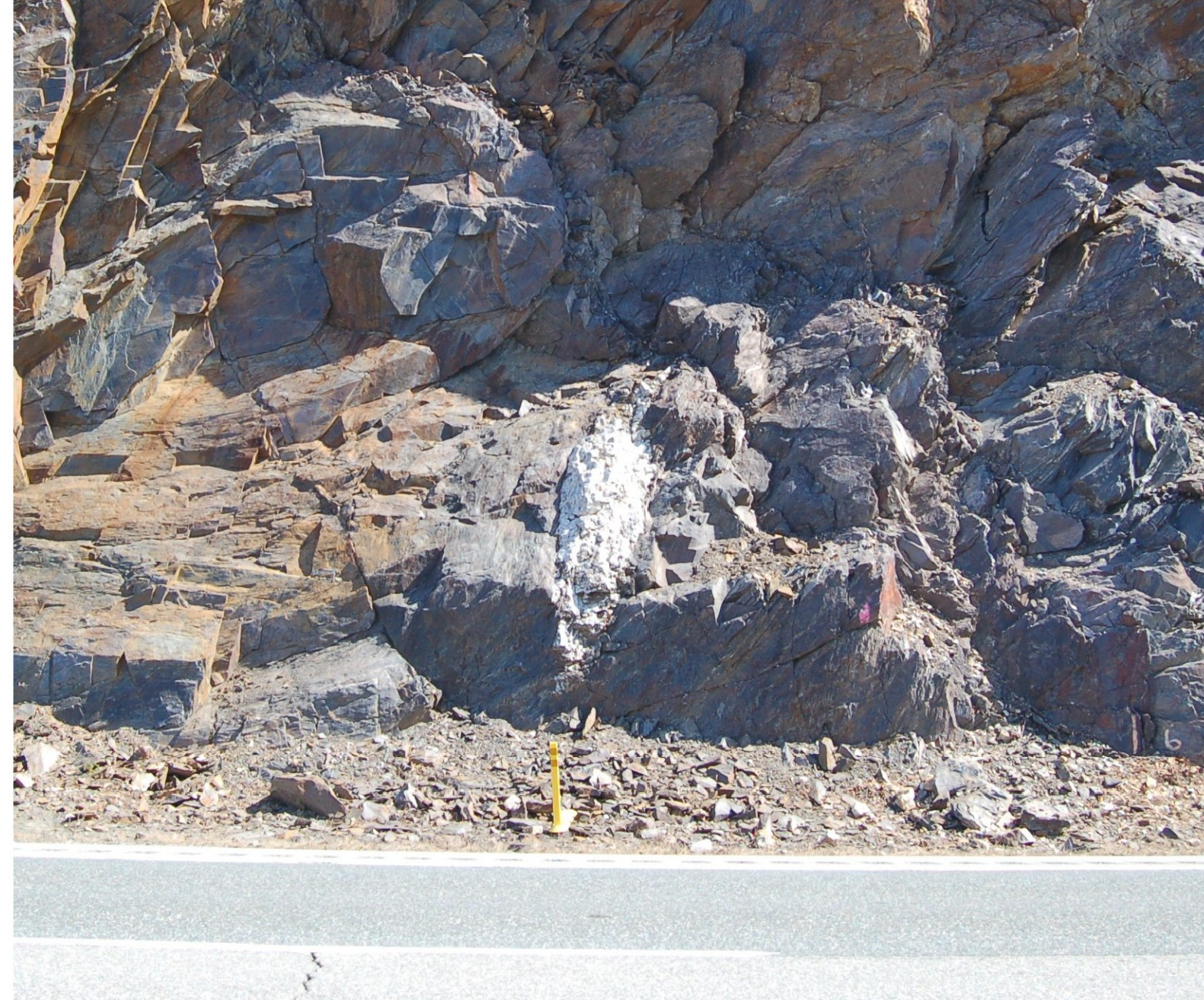
STA. 1849+50 MACHINE SCALING AT TOP ONLY
