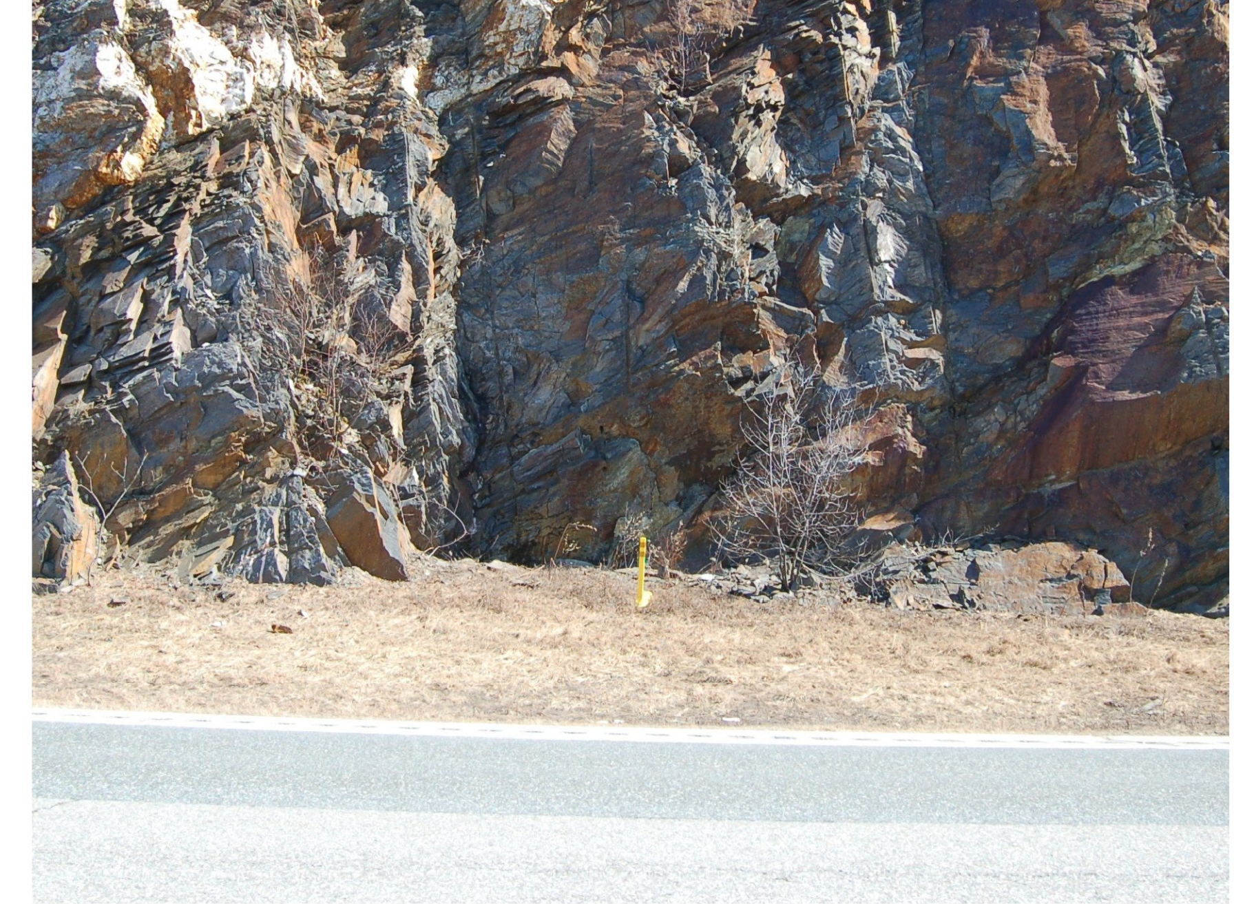
STA. 1857+00 MACHINE SCALING AT TOP ONLY
