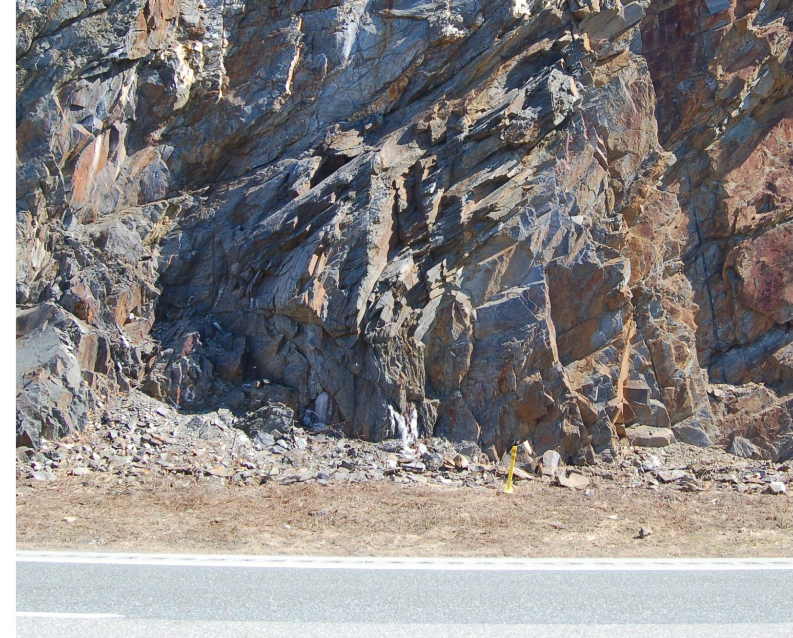
STA. 1851+00 MACHINE SCALING AT TOP ONLY
