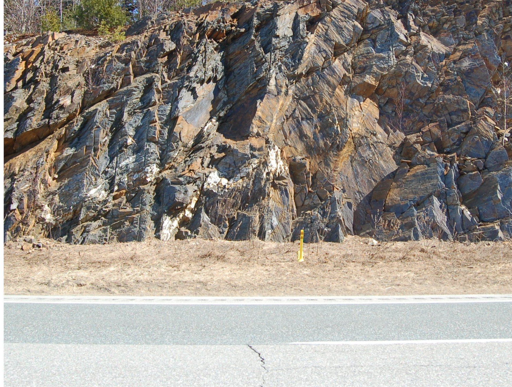
STA. 1858+00 MACHINE SCALING AT TOP ONLY
