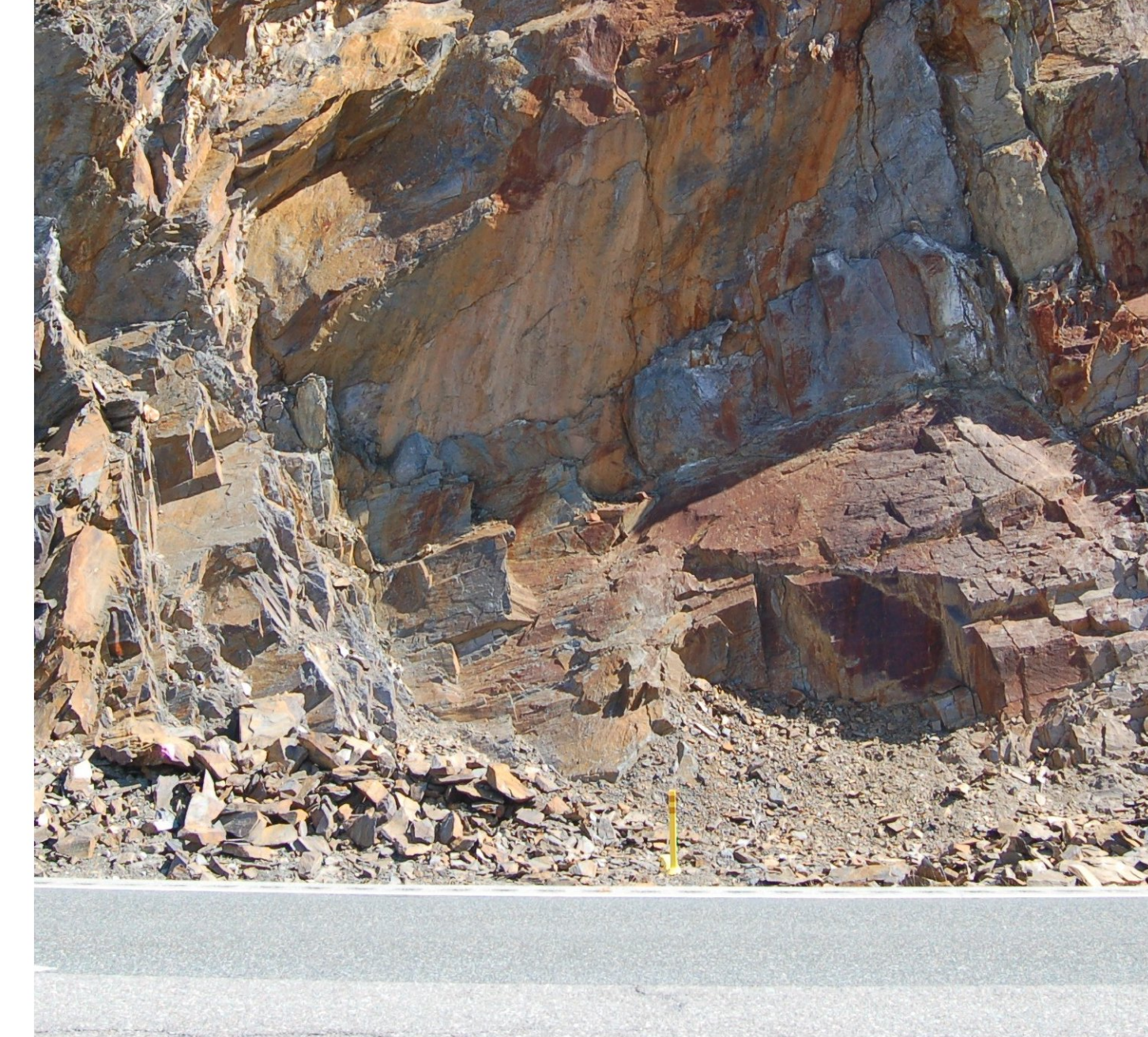
STA. 1853+00 MACHINE SCALING AT TOP ONLY
