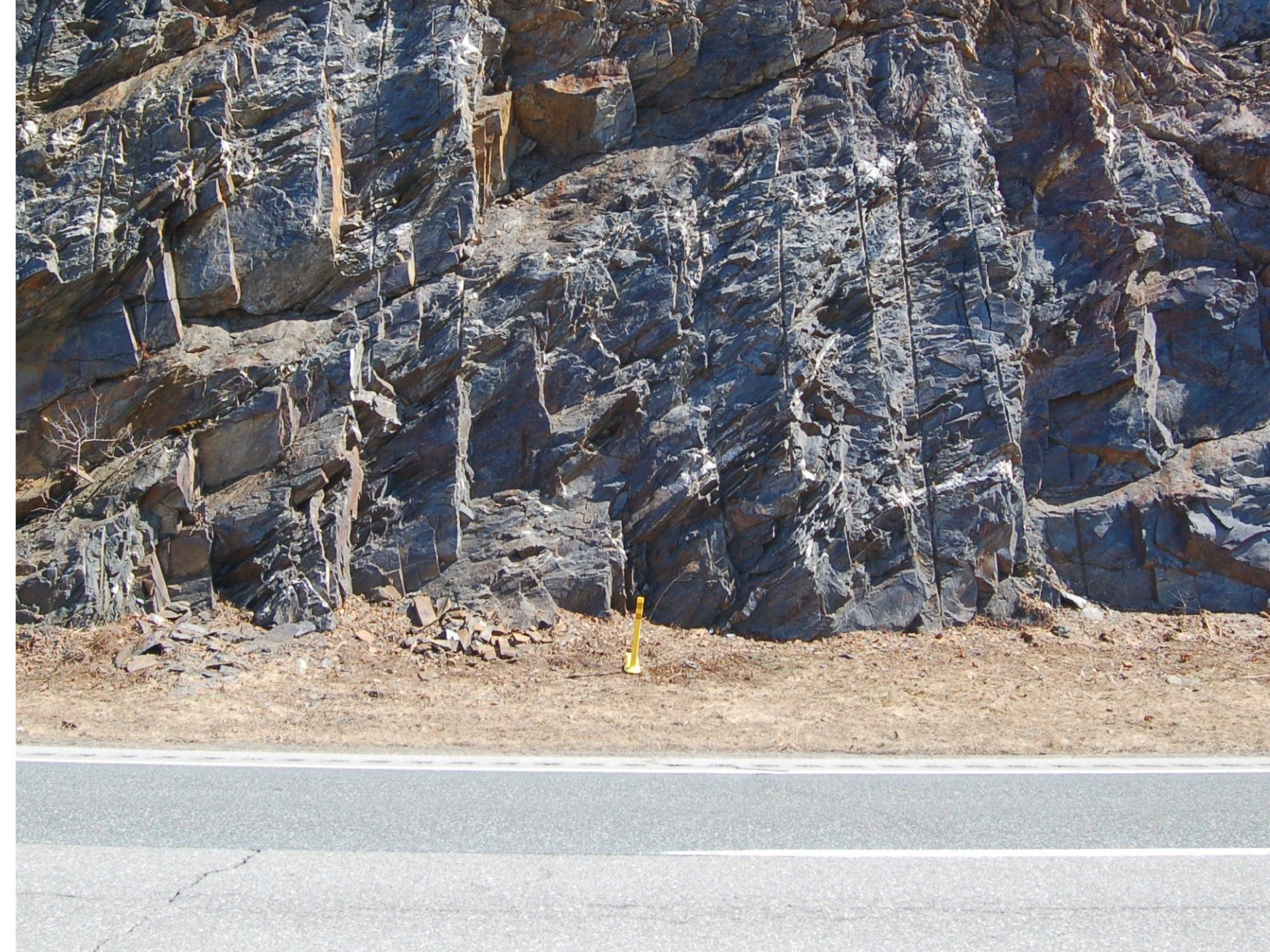
STA. 1848+00 MACHINE SCALING AT TOP ONLY
