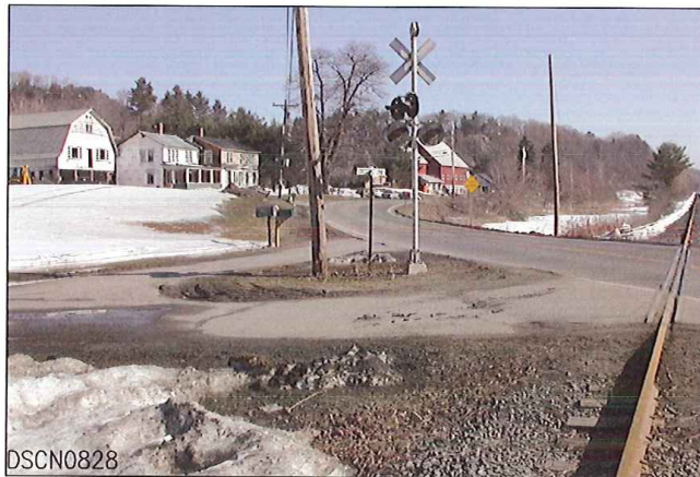
LOOKING FROM SOUTH TO WEST
