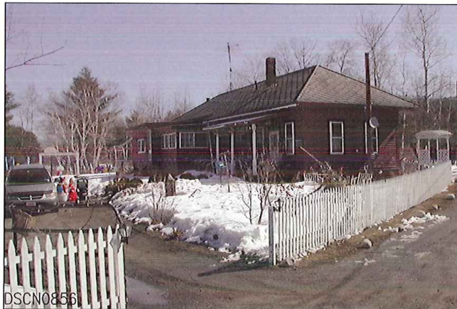
LOOKING FROM WEST TO NORTH
