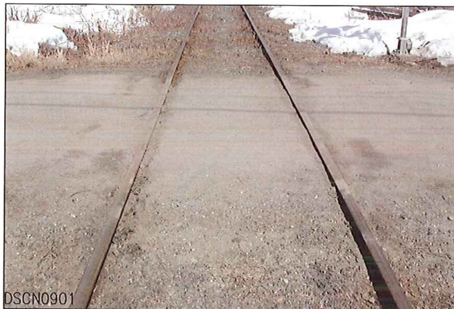
LOOKING FROM SOUTH TO NORTH
