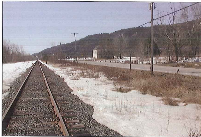
LOOKING FROM SOUTH TO WEST
