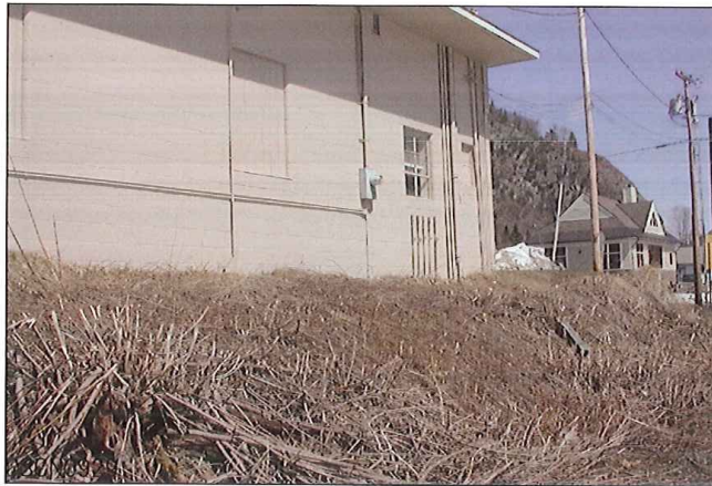
LOOKING FROM SOUTH TO WEST
