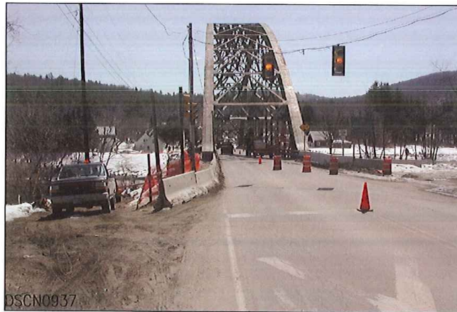
BRIDGE EAST OF CROSSING
