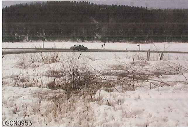
LOOKING FROM NORTH TO WEST
