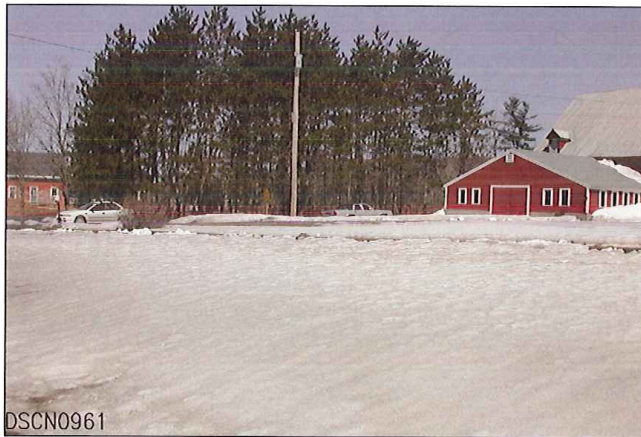
LOOKING FROM SOUTH TO EAST
