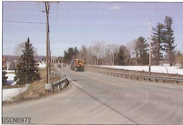
LOOKING FROM WEST TO NORTH
