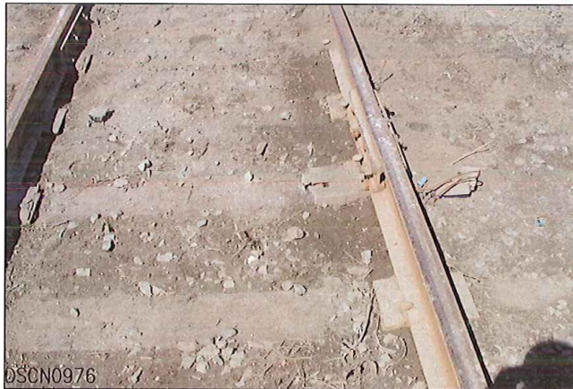
SOUTH SIDE OF CROSSING
