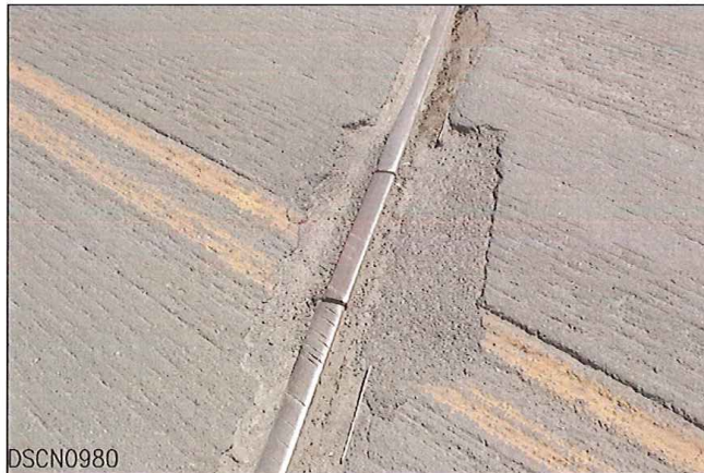
SHORT RAIL REPAIR - EAST RAIL
