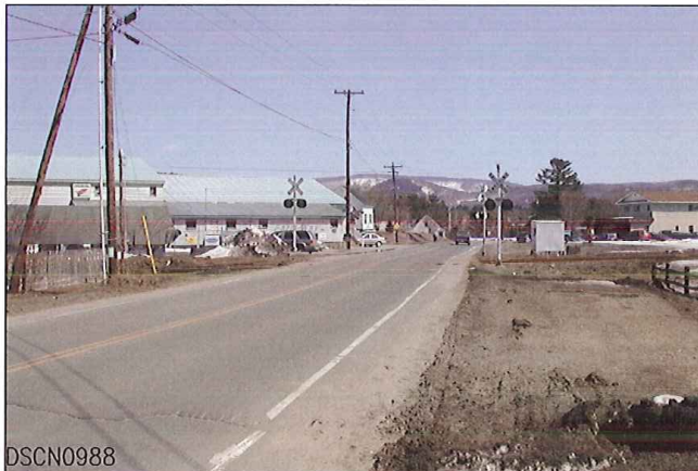
LOOKING FROM WEST TO EAST
