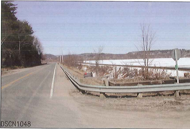
LOOKING FROM WEST TO NORTH
