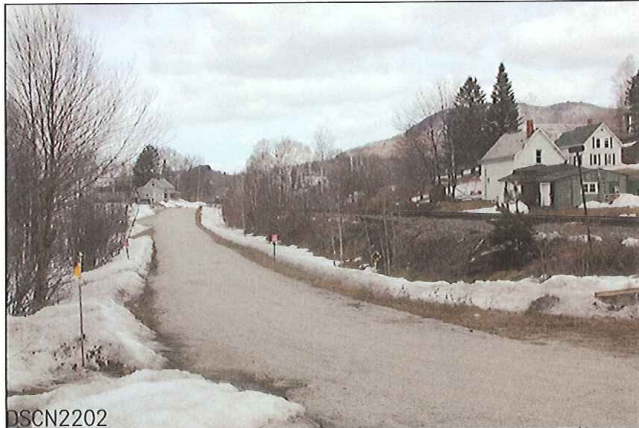
LOOKING FROM WEST TO NORTH
