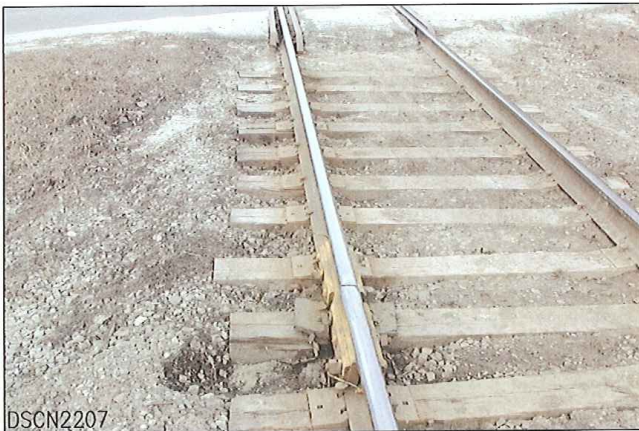
LOOKING FROM SOUTH TO NORTH
