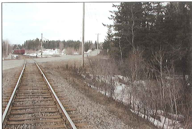
LOOKING FROM SOUTH TO EAST
