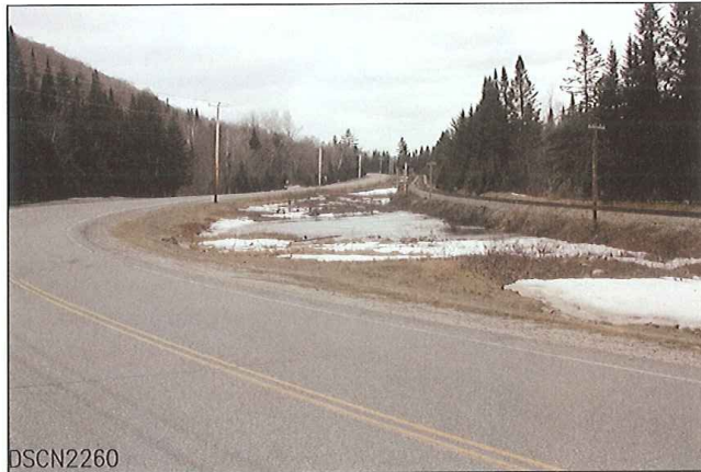
LOOKING FROM WEST TO EAST
