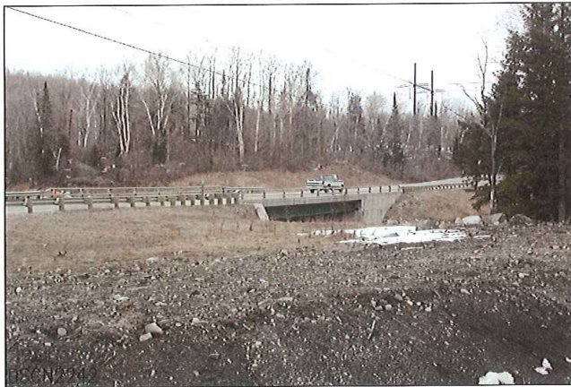
LOOKING FROM SOUTH TO EAST
