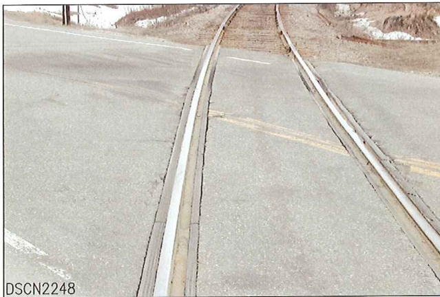
LOOKING FROM SOUTH TO NORTH
