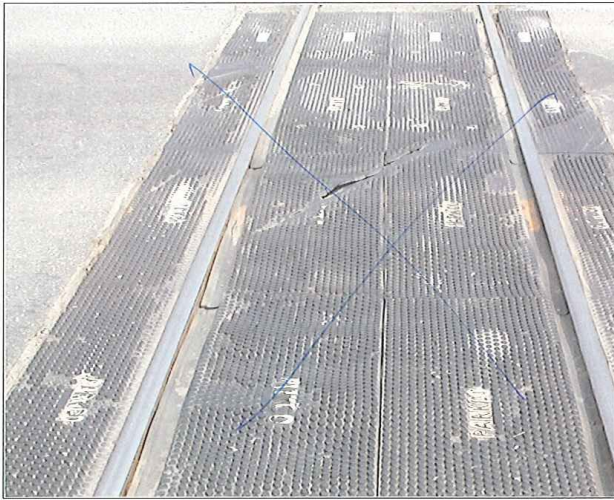
Damaged Rubber Crossing
