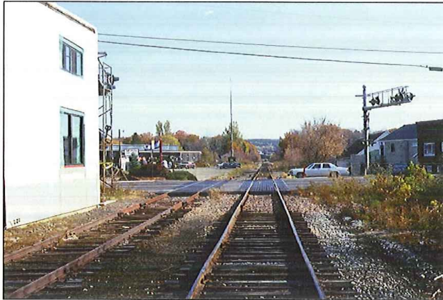
LOOKING EAST MAINLINE ON RIGHT SIDE
