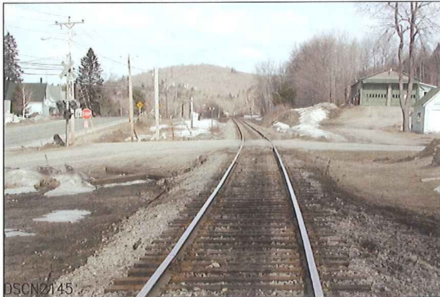
LOOKING FROM SOUTH TO NORTH
