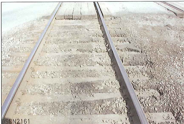
LOOKING FROM SOUTH TO NORTH - MAINLINE TRACK
