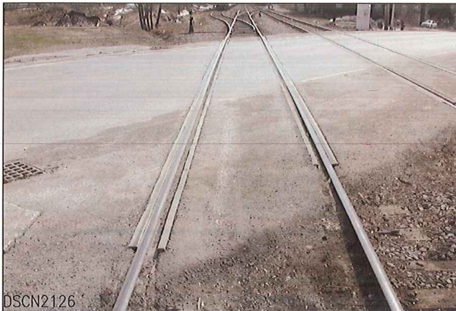
LOOKING FROM NORTH TO SOUTH SIDETRACK
