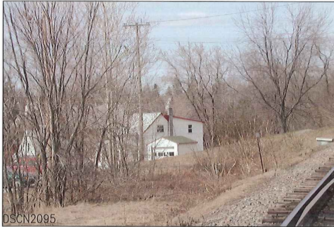
LOOKING FROM SOUTH TO WEST
