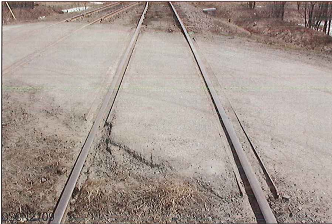
LOOKING FROM NORTH TO SOUTH MAINLINE
