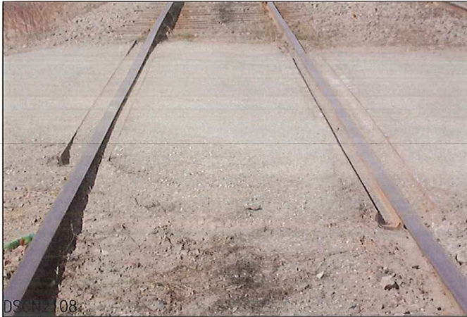
LOOKING FROM SOUTH TO NORTH MAINLINE
