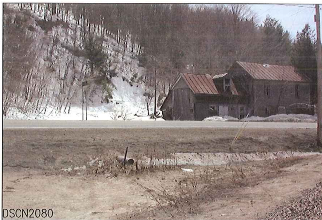
LOOKING FROM SOUTH TO WEST
