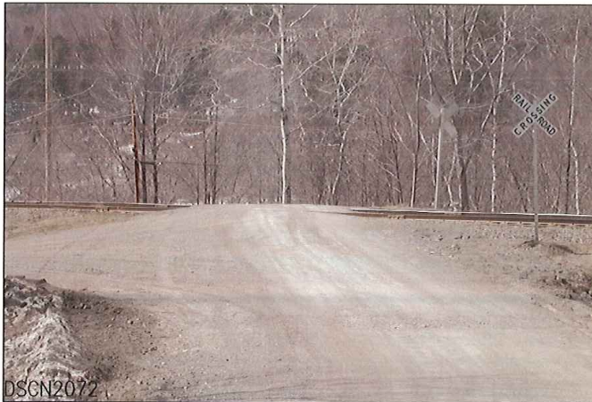
LOOKING FROM WEST TO EAST
