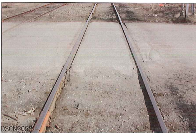
LOOKING FROM NORTH TO SOUTH – MAINLINE
