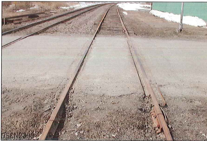
LOOKING FROM SOUTH TO NORTH – SIDE TRACK
