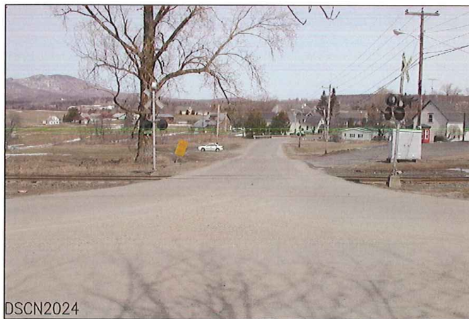
LOOKING FROM WEST TO EAST
