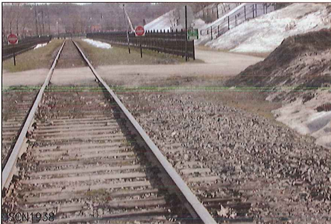
LOOKING FROM NORTH TO WEST
