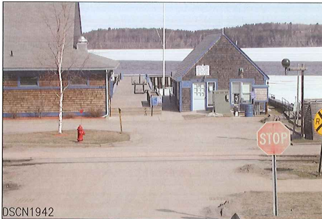
LOOKING FROM WEST TO EAST
