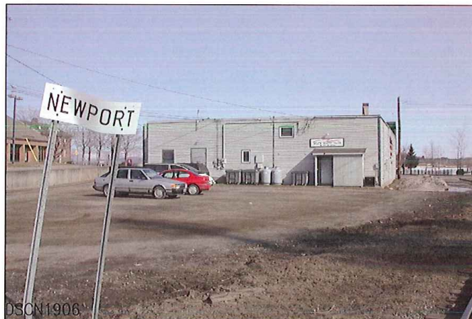
LOOKING FROM SOUTH TO WEST
