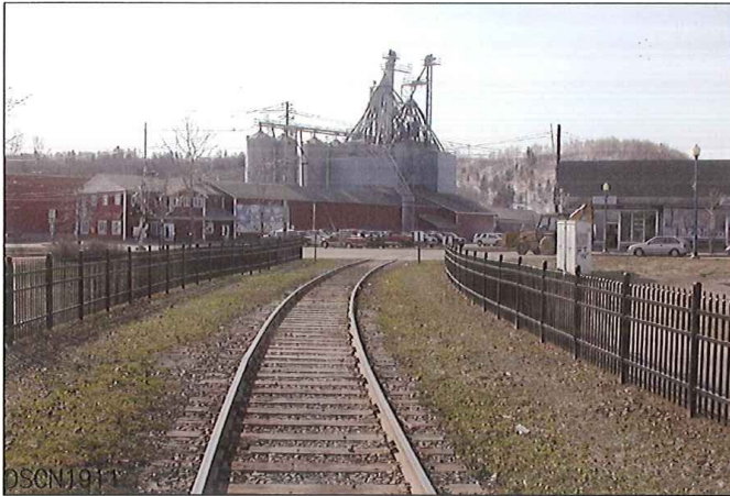
LOOKING FROM NORTH TO SOUTH – MAINLINE
