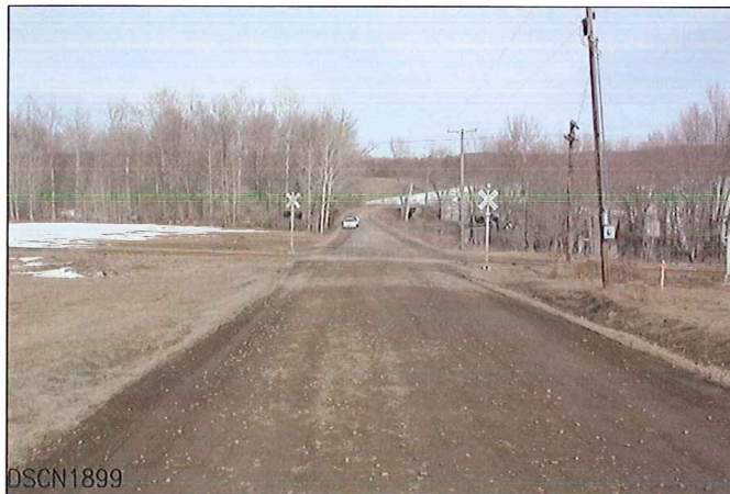
LOOKING FROM WEST TO EAST
