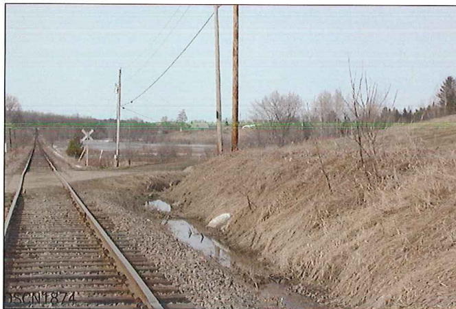
LOOKING FROM SOUTH TO EAST
