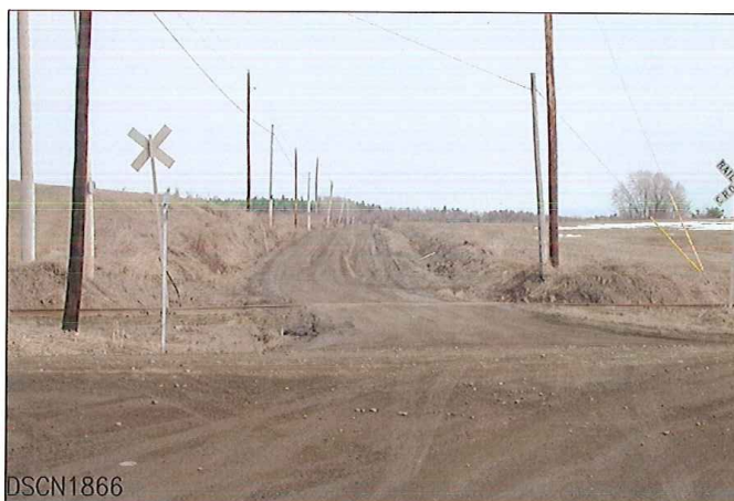
LOOKING FROM WEST TO EAST
