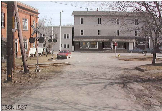
LOOKING FROM WEST TO EAST
