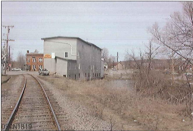
LOOKING FROM SOUTH TO EAST
