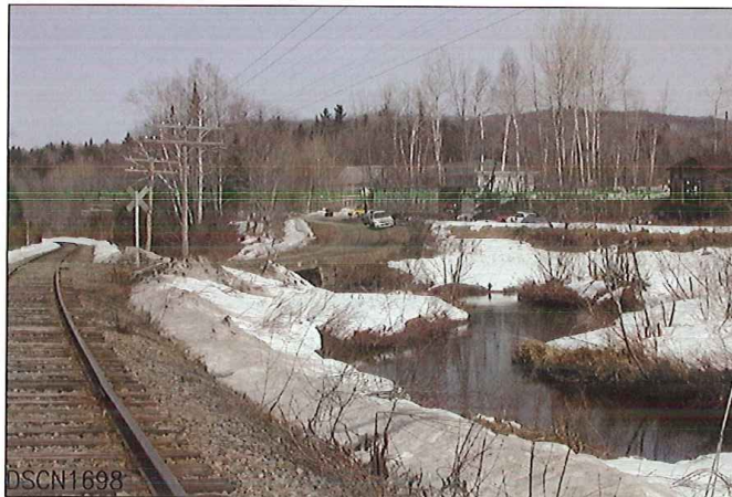
LOOKING FROM SOUTH TO EAST
