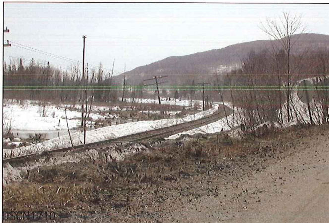
LOOKING FROM WEST TO SOUTH
