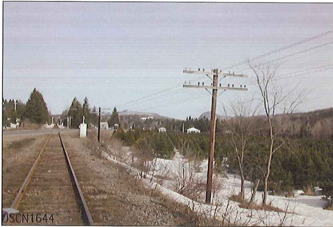
LOOKING FROM SOUTH TO EAST
