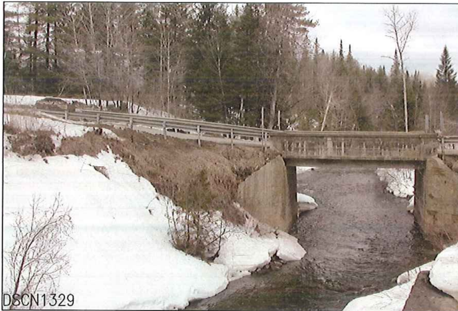
LOOKING FROM SOUTH TO WEST
