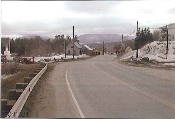
LOOKING FROM WEST TO EAST
