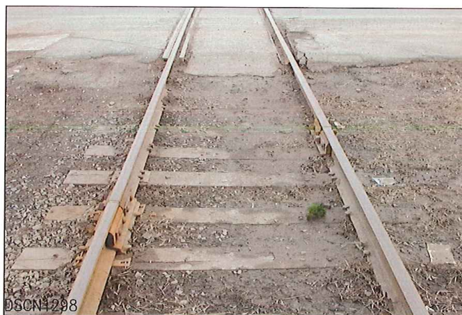
LOOKING FROM SOUTH TO NORTH
