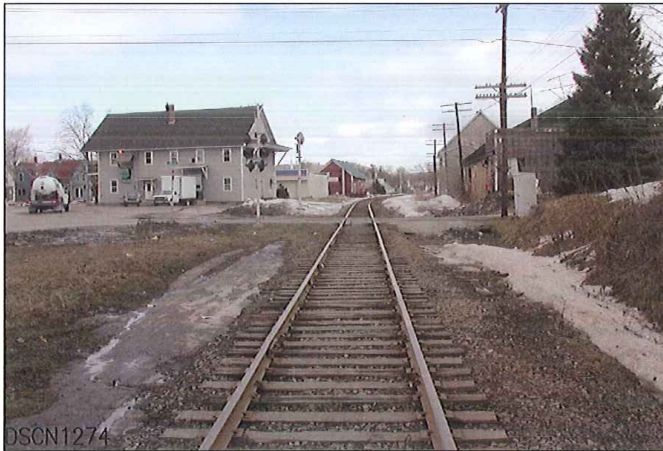
LOOKING FROM SOUTH TO NORTH
