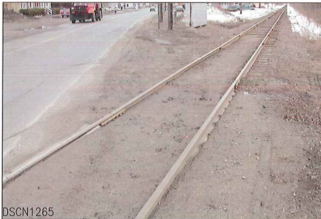
SOUTH SIDE OF CROSSING
