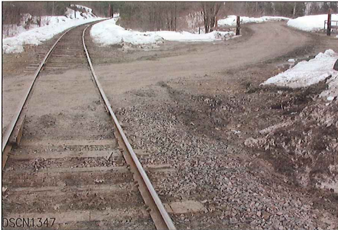
LOOKING FROM SOUTH TO NORTH
