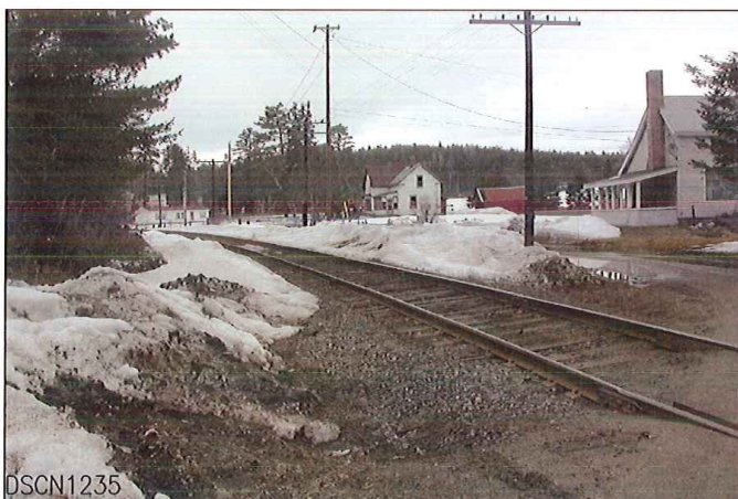
LOOKING FROM WEST TO NORTH
